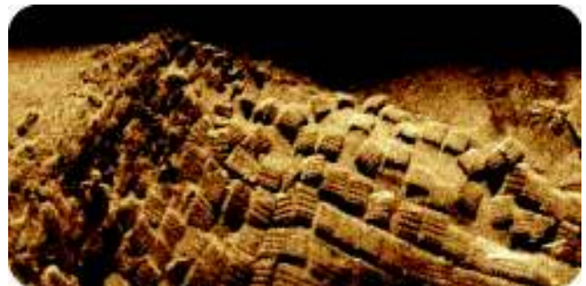
Sunken concrete blocks at Świnoujście Harbour, Poland. (courtesy of M. Szatan)
